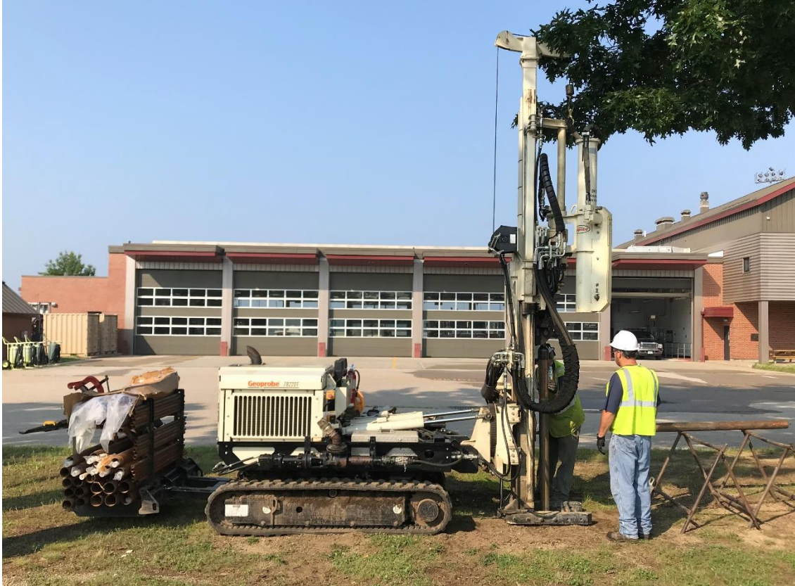
Direct push soil investigation
