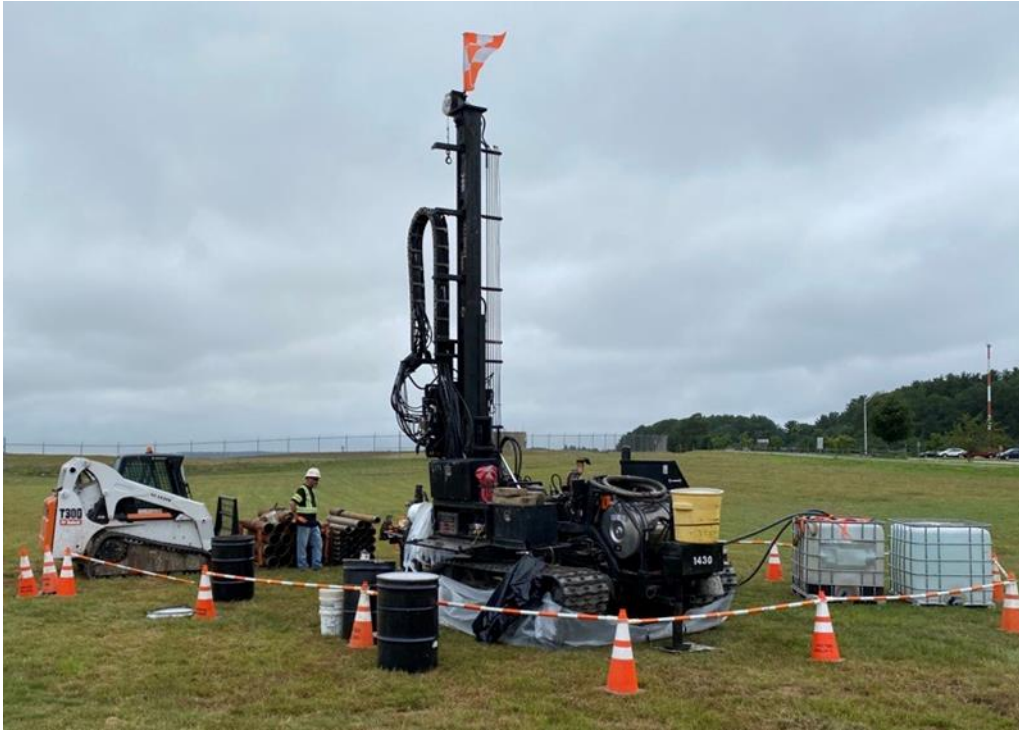
Monitoring well installation
